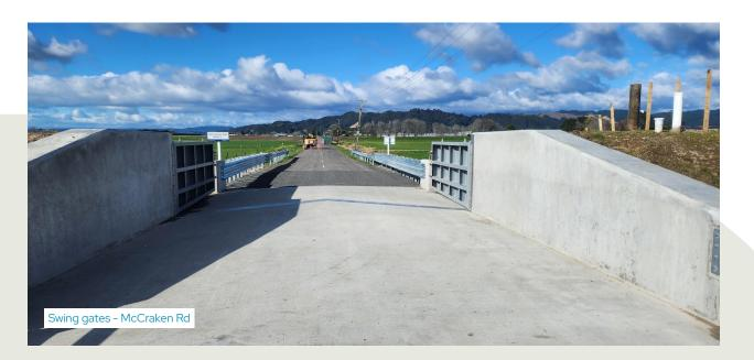
In a flood event, these swing gates will act as a barrier on the road, keeping cars from entering a flood zone, and maintain the stopbank height of the Floodway, creating a channel that will help send water out to the Rangitāiki River mouth.
