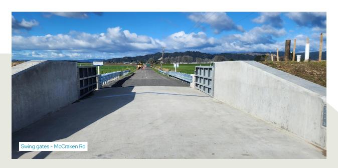
In a flood event, these swing gates will act as a barrier on the road, keeping cars from entering a flood zone, and maintain the stopbank height of the Floodway, creating a channel that will help send water out to the Rangitāiki River mouth.
