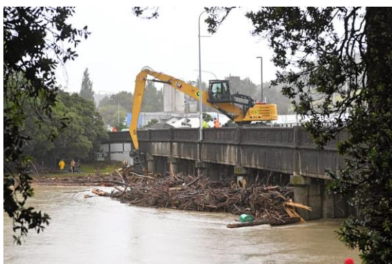
Figure A37. Woody debris removal during flood.
