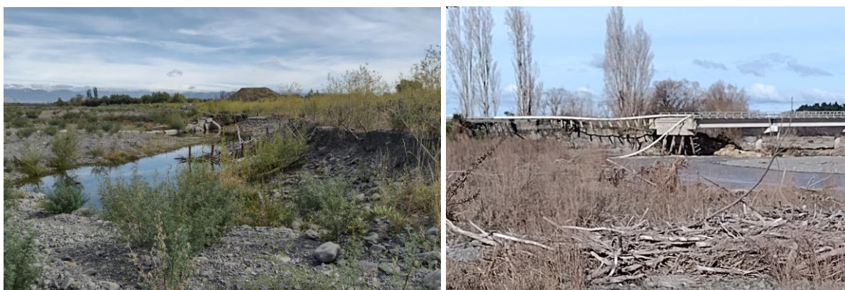
Figure 16. Bank erosion with damaged Akmon & rope/rail groynes (left). SH50 Bridge wash out (right).
