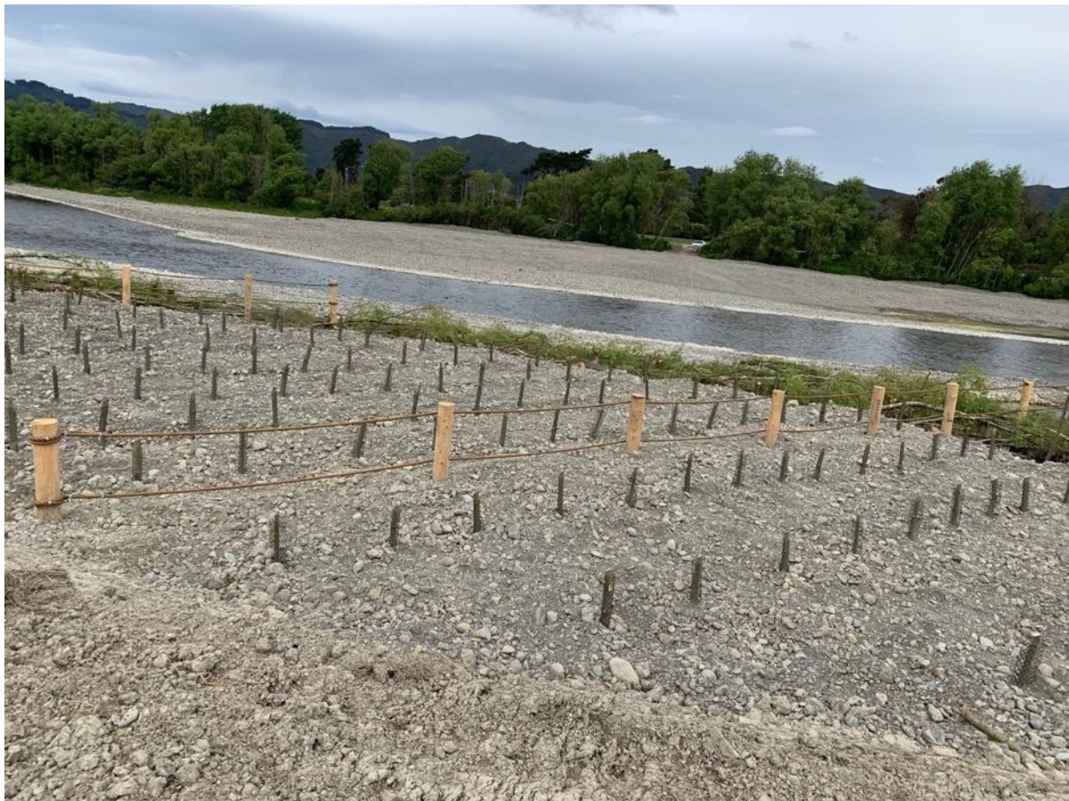
Figure 1-1 Erodible buffers being established on Te Awa Kairangi (Hutt River)
